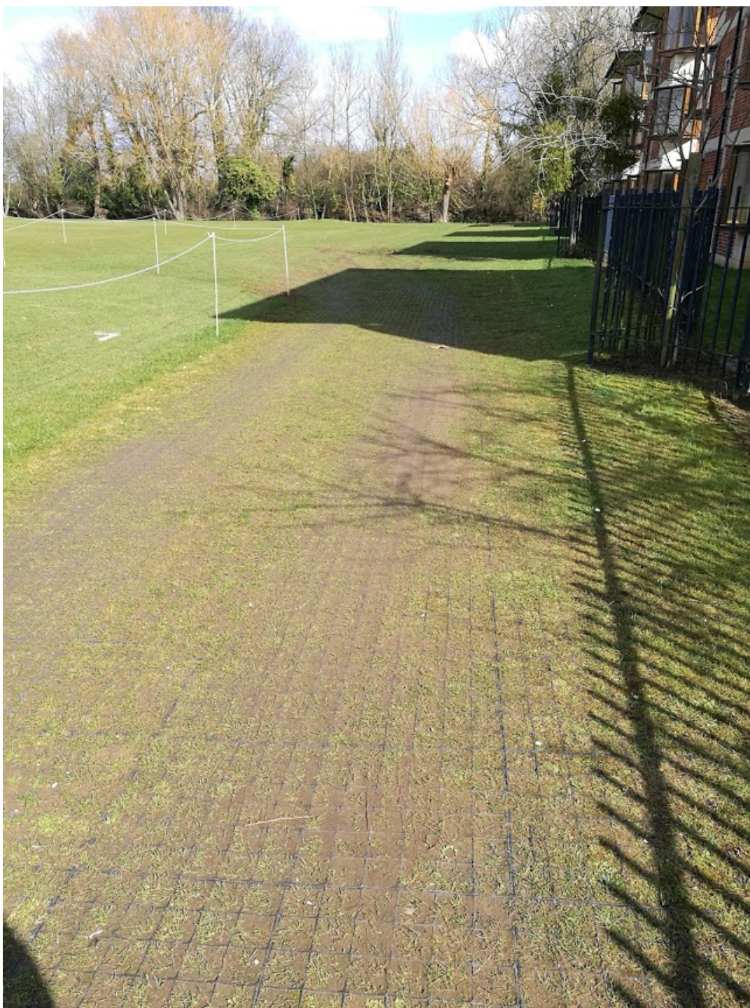
Continuation of existing access onto the field, showing existing surfacing, and location of new Formalised access.
